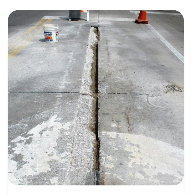
Precise Patch of Ohio, repaired a crumbling, moving street joint that they hoped would last through a frigid, Lake Erie winter of ice, snow, street traffic and snow plows.
